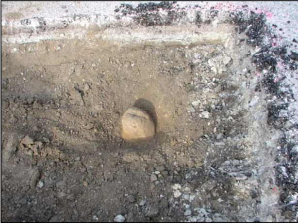
Corner stone - view from East.
