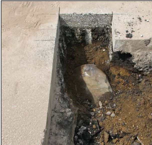
Corner stone - overhead view from south, showing top of stone after hole was refilled and a new area cut out above stone.
