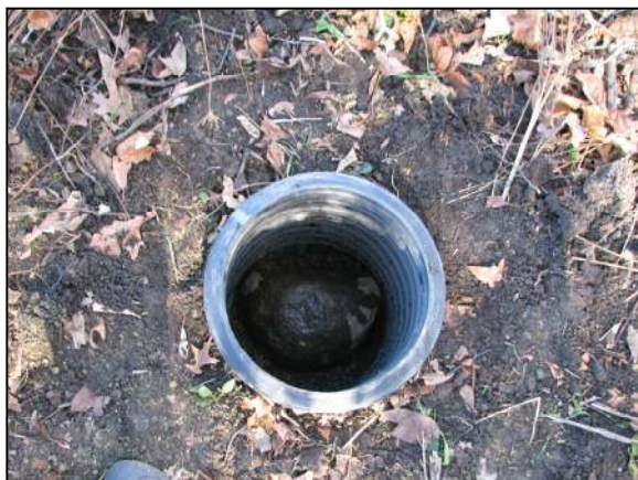
The stone within the section of HDPE storm pipe, immediately prior to being encased in concrete.
