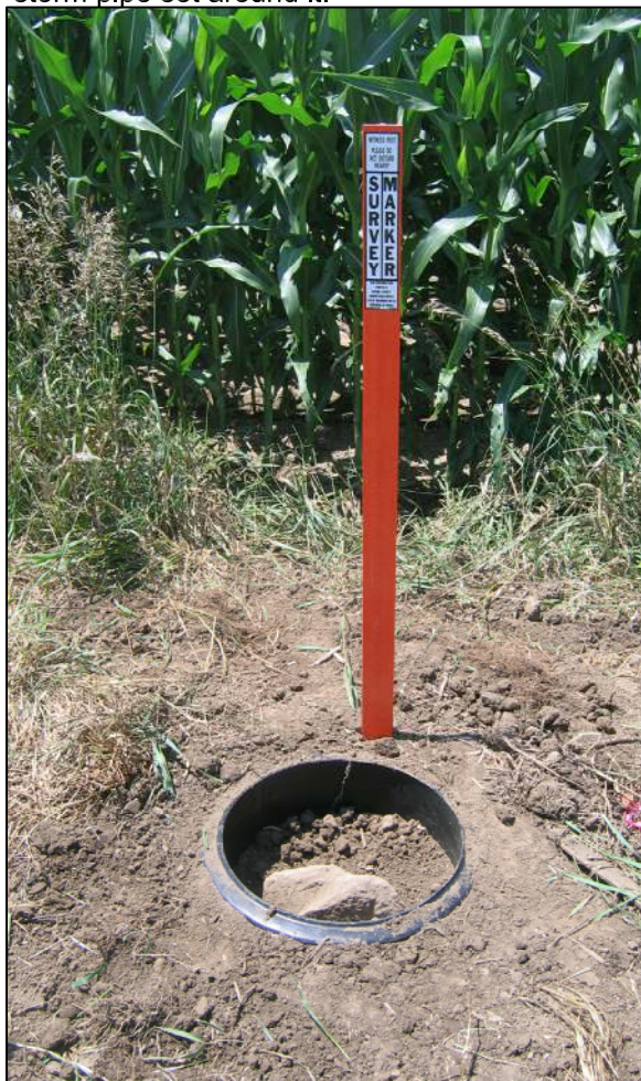
The stone with the vertical section of plastic storm pipe set around it.
