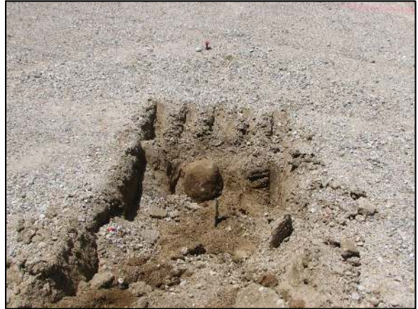
The first stone found (not held) and the rebar.
