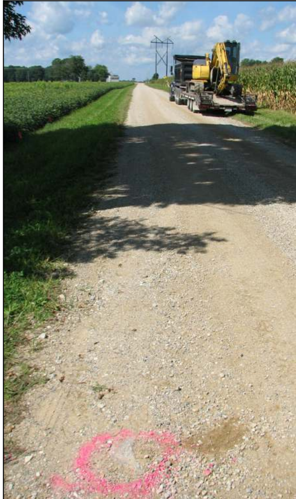
The top stone, visible at the surface of the road. View of County Road 950 North to the west.
