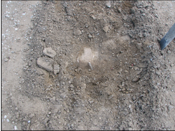
View of the stone and bent rebar from the north and above.
