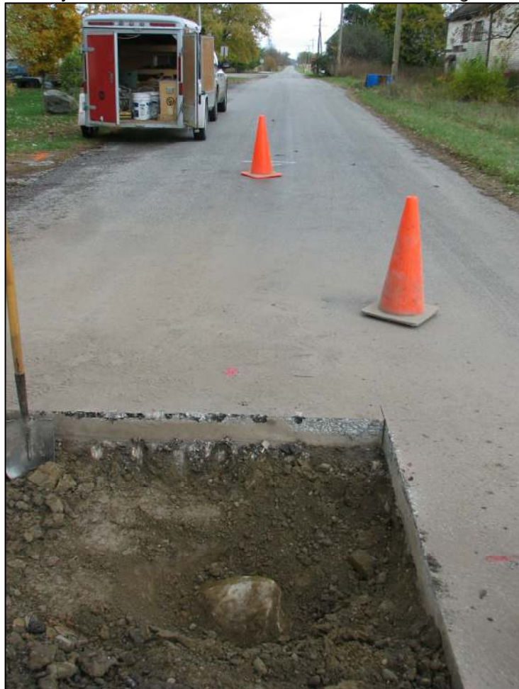
View from the west looking across the stone and east along County Road 300 North. U.S. 421 crosses in the foreground.
