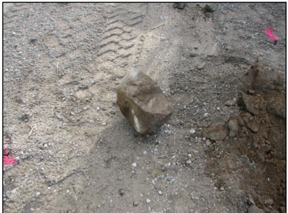
View of the stone removed from the road bed.
