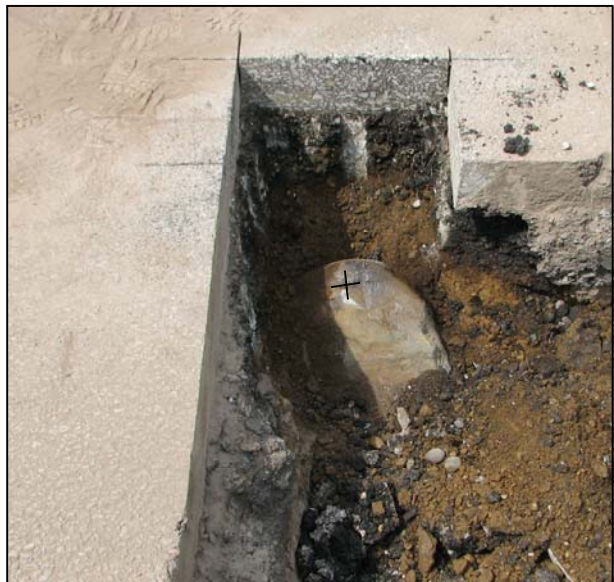
Same view as to left, with chiseled "+" on the top of the stone enhanced for ease of visual detection.
