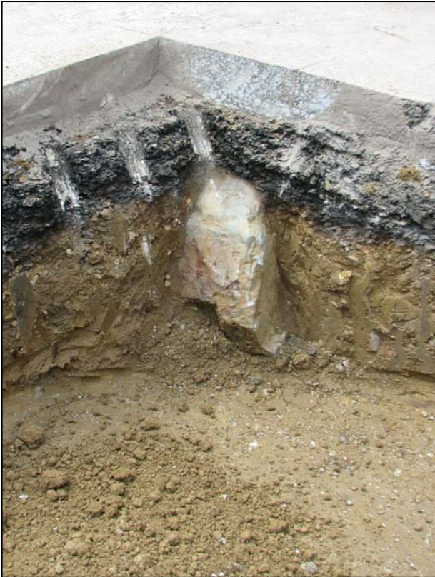
Corner stone - view of south half of stone, exposed in corner of hole, from southeast.
