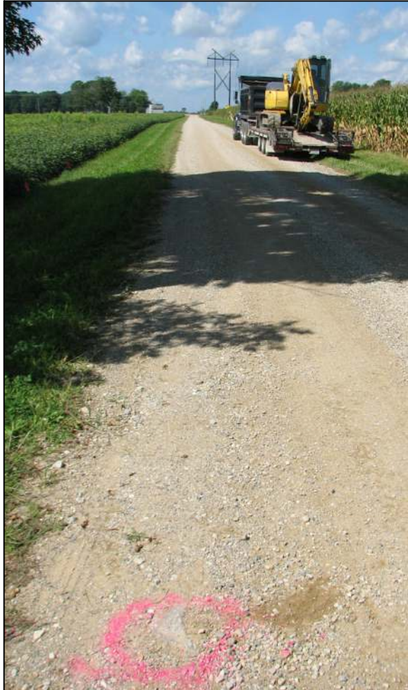
The top stone, visible at the surface of the road. View of County Road 950 North to the west.
