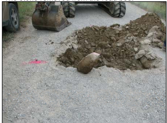
The stone removed from the road bed.
