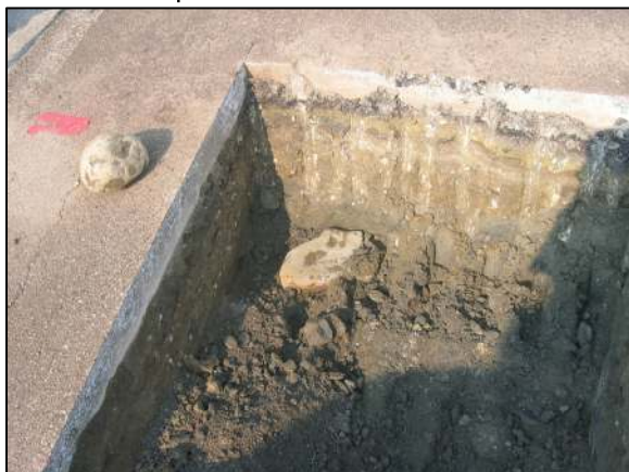
The lower stone as stood up, after the area of excavation was filled back to the level of the original bottom of the road bed.
