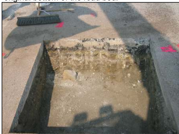
The lower stone as stood up, after the area of excavation was filled back to the level of the original bottom of the road bed.
