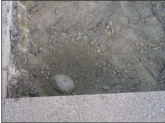
The lower stone as found, apparently on its side. Note that the bottom of the road bed is above the top of the stone.
