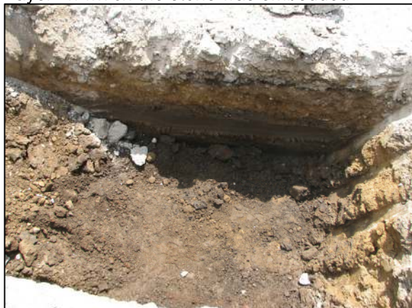
Excavation below the stone, showing the cross section of the roadway. Note the distinct clay layer in which the stone was embedded.
