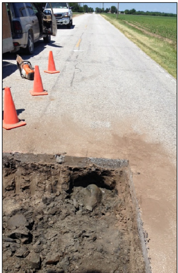
View from the south, looking across the stone and north along County Road 150 West.
