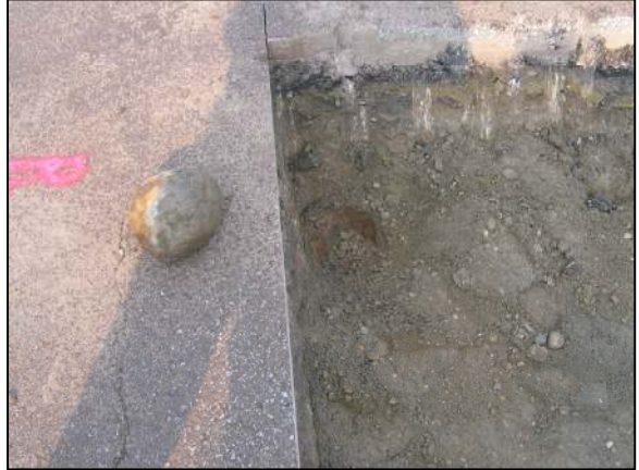
The lower stone as stood up. Note that the top of the stone protrudes a few inches into the bottom of the road bed when stood up.
