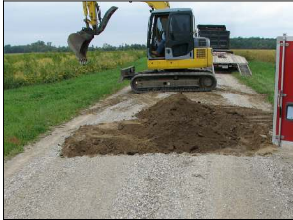
Excavation at the subject corner on 9/11/2014
