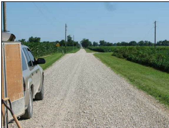
View prior to excavation, looking north along Meridian Road from above the closing corner.
