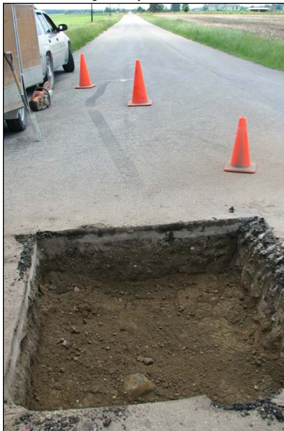
View from the north, looking across the stone (stood up and partially repacked in fill material) and south along County Road 550 East.
