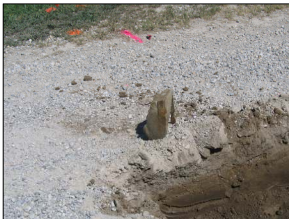
The stone, removed from the clay below the road bed and stood up in the orientation in which it was found.
