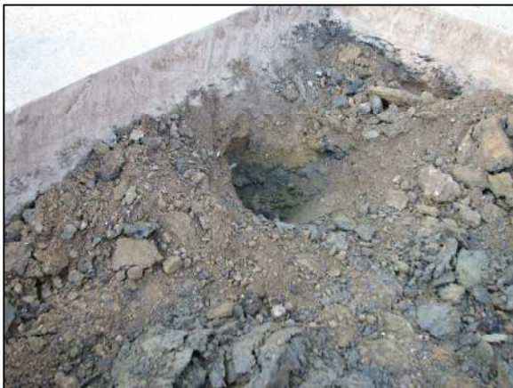
The hole from which the stone was removed, demonstrating that the stone was embedded in the clay layer below the road bed.
