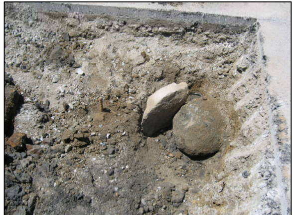
All four found monuments. The rebar, rail and lower stone are undisturbed. The upper stone is reset in the approximate position as found.
