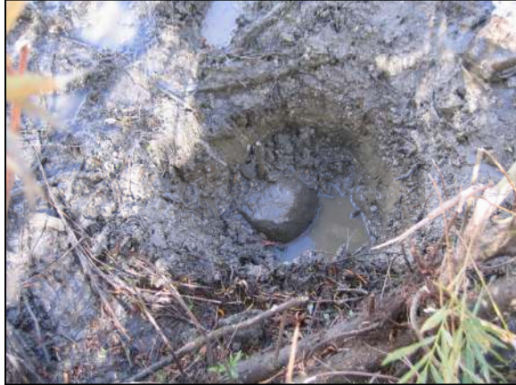
The stone and rebar as exposed on 10/7/2009.
