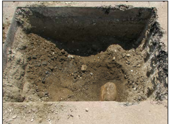
The stone at the Hamilton County corner (corner 2).
