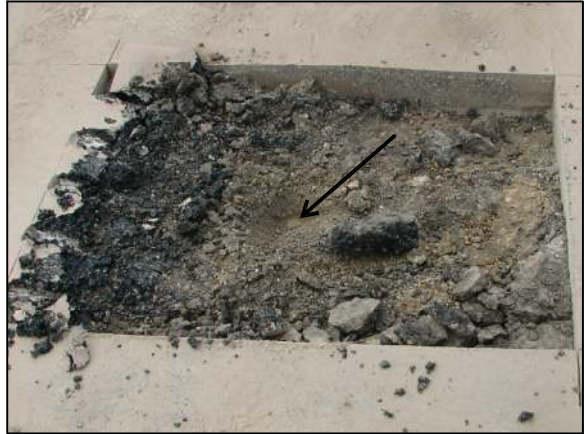
The top of the boat spike found driven into the stone at the Hamilton County corner (corner 2).
