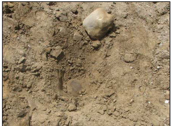
The upper stone removed from the road bed and the lower stone embedded in the road bed.
