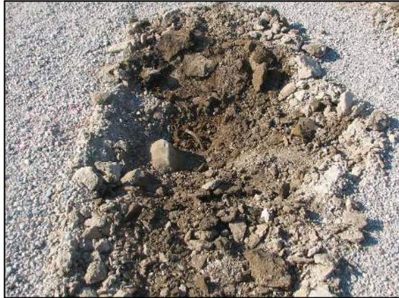
The stone and rebar as originally exposed.
