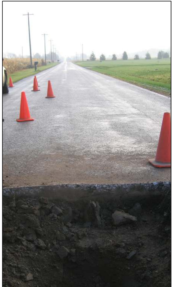
View from above the stone, looking east along County Road 100 South.
