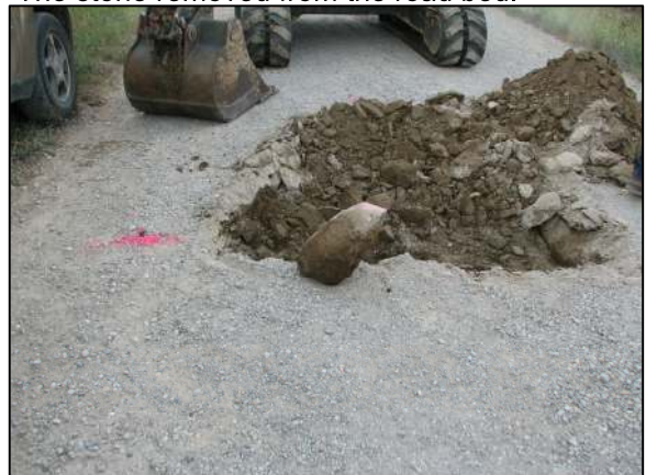
The stone removed from the road bed.
