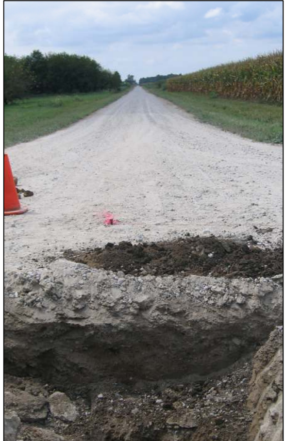
View from above the stone, looking west along County Road 400 North.
