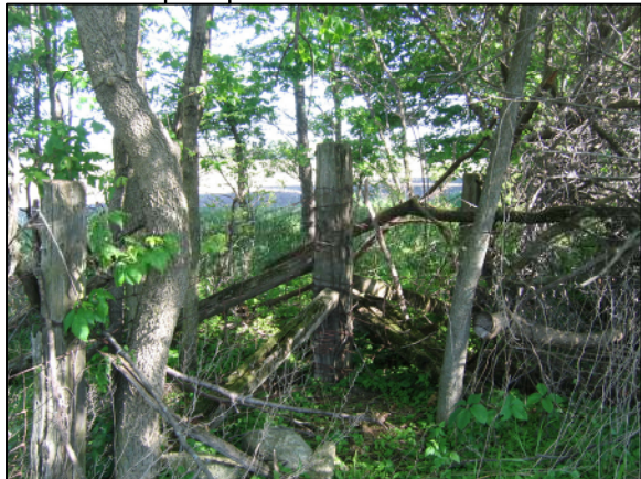
The corner post prior to excavation.
