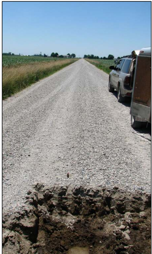
View from the north looking across the stone and south along County Road 300 West.
