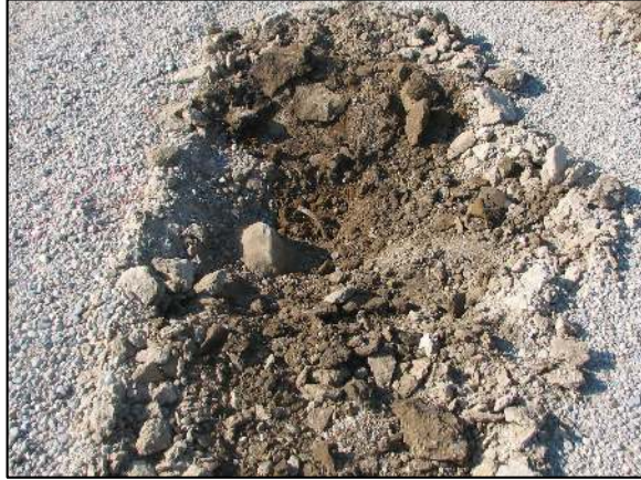
The stone and rebar as originally exposed.
