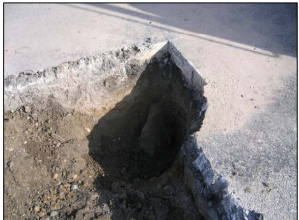
Similar view to above. View from the southwest.
