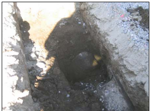
The stone from above and east.
