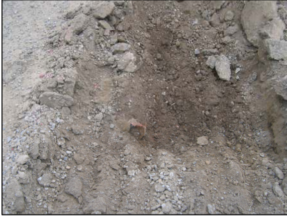
The top of the railroad rail, as found.
