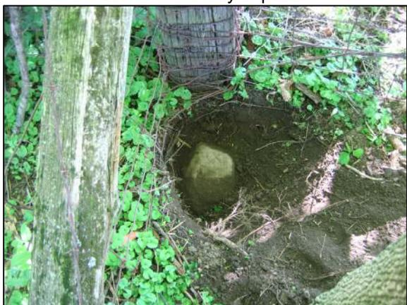
A vertical section of plastic storm pipe set around the stone. The stone was left as found, but surrounded by the section of storm pipe.
