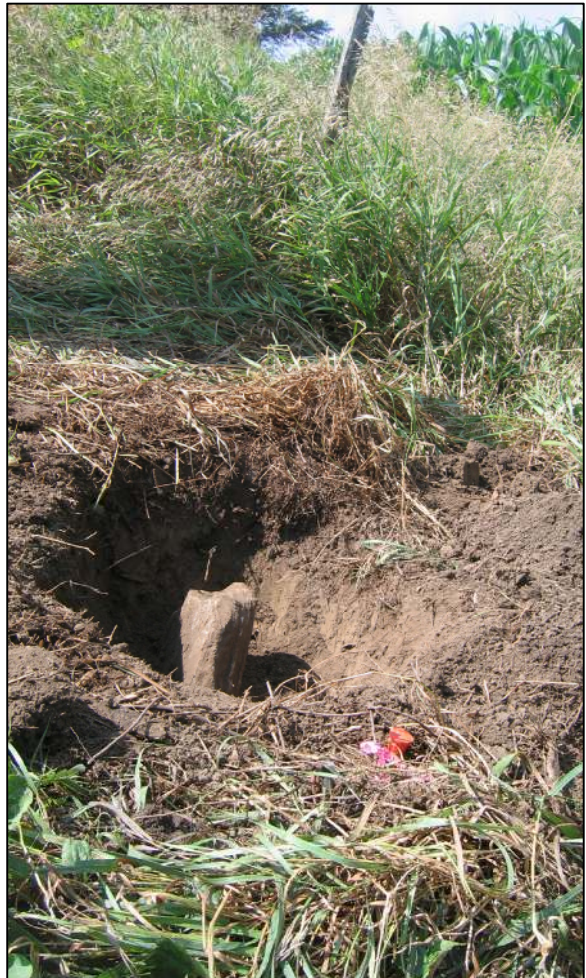
View from the north, showing the stone, rebar and a remaining post of the north-south fence.
