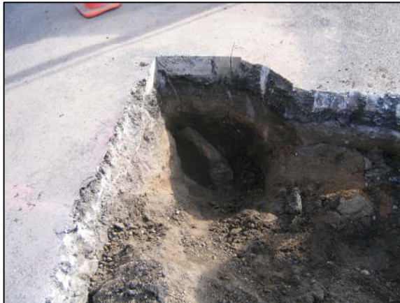
View of the stone more fully exposed. View from the west.
