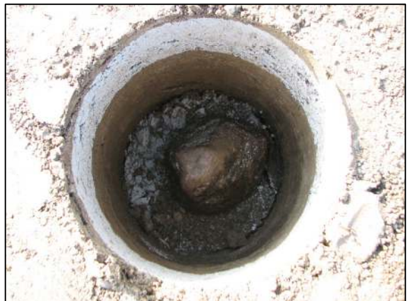
The stone from above shortly before being encased in concrete as part of setting the harrison monument over the stone.
