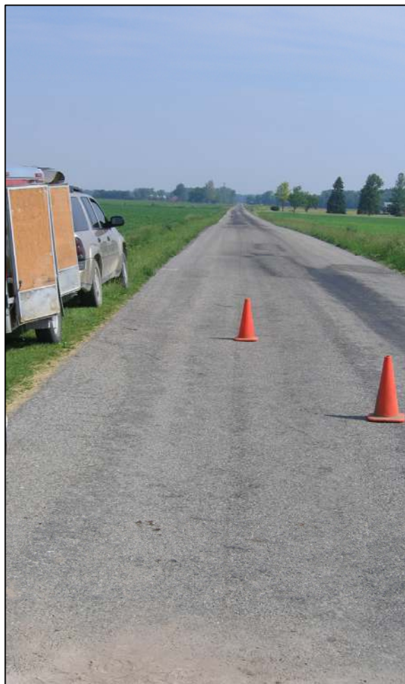
View from above corner 2, looking north along County Road 600 East.
