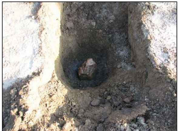
The stone from above shortly before being encased in concrete as part of setting the harrison monument over the stone.
