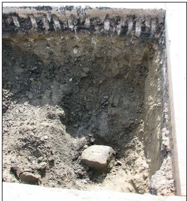
Overhead view from West.
