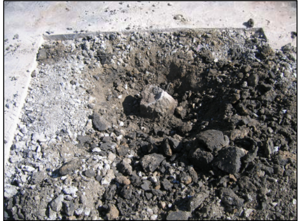
View of the stone at the closing corner (corner 2) as first exposed.
