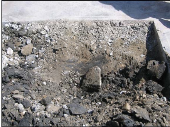
View of the stone at the standard corner (corner 1) as first exposed.
