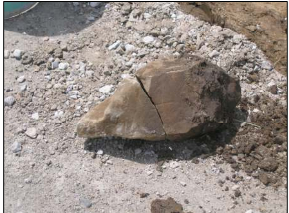
The two parts of the stone removed from the road bed. The side facing the camera was the west side and the "sharp point" on the top of the rock is on the left in this picture.
