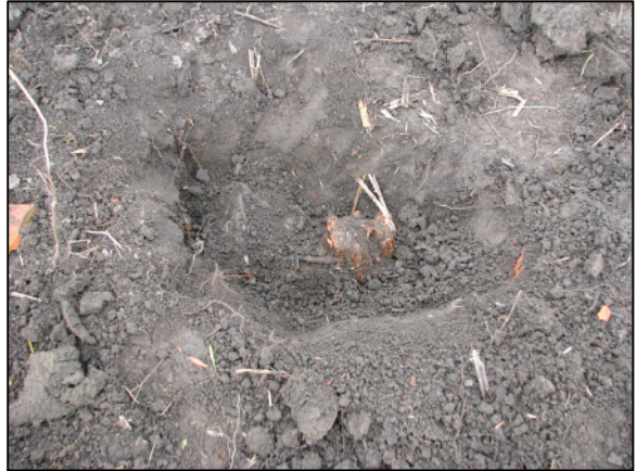
The base of the corner post as found and uncovered in December 2012.
