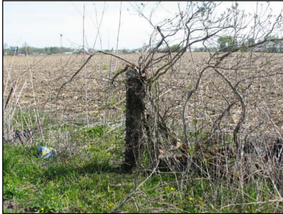
The old corner post as found in April 2012.
