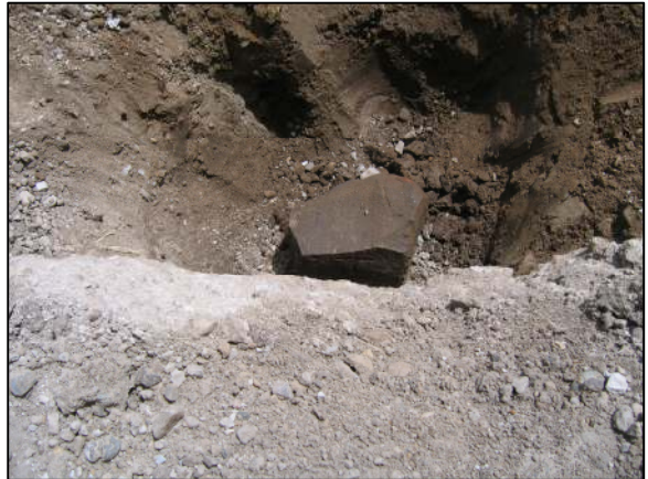
The bottom part of the stone found embedded in the road. Not the etched + on the side.
