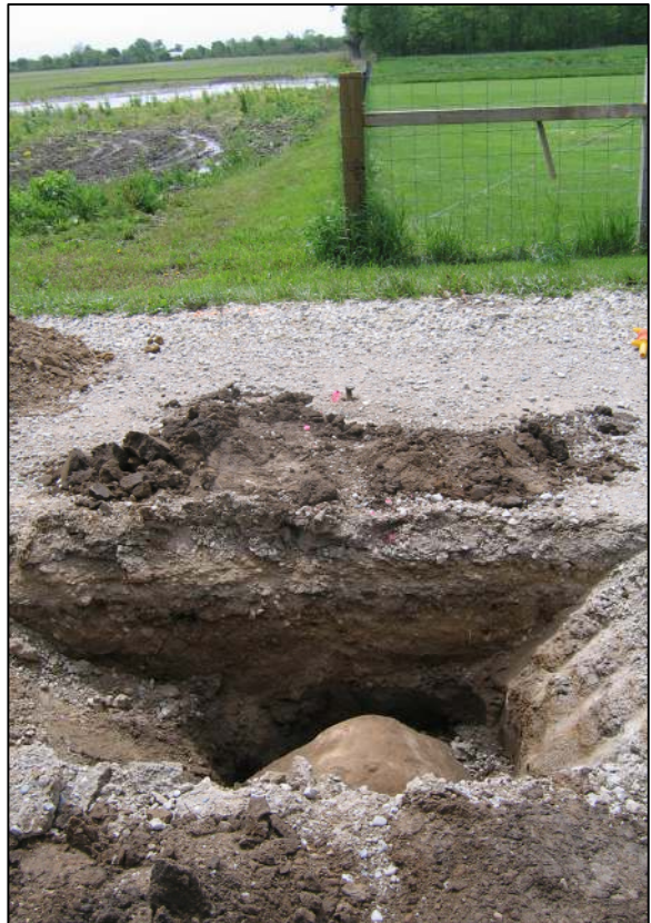
View from the north, looking across the stone and south along the fence to the south.
