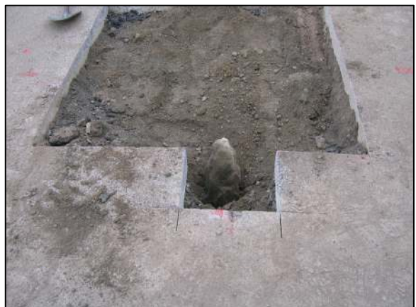
The stone, temporarily put back in the road bed and stood in vertical orientation.
