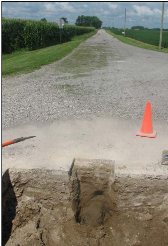
View from the west looking across the lower stone and west along County Road 50 South.
