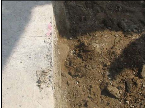
The upper stone as it was originally exposed.
