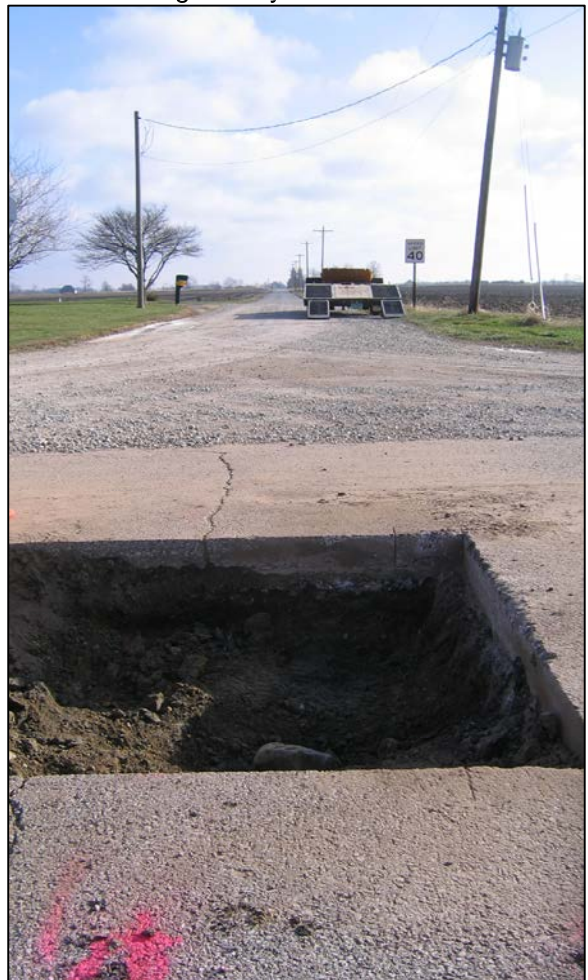
View from the west, looking across the stone and east along County Road 650 South.
