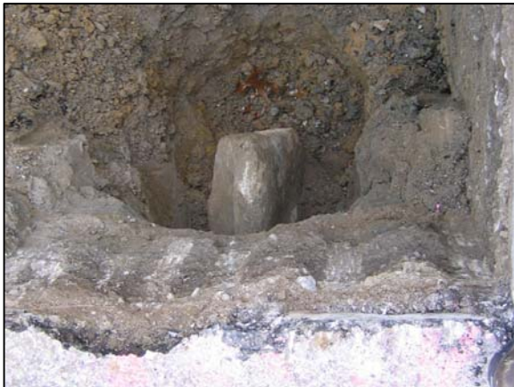
Corner stone. View from above.
