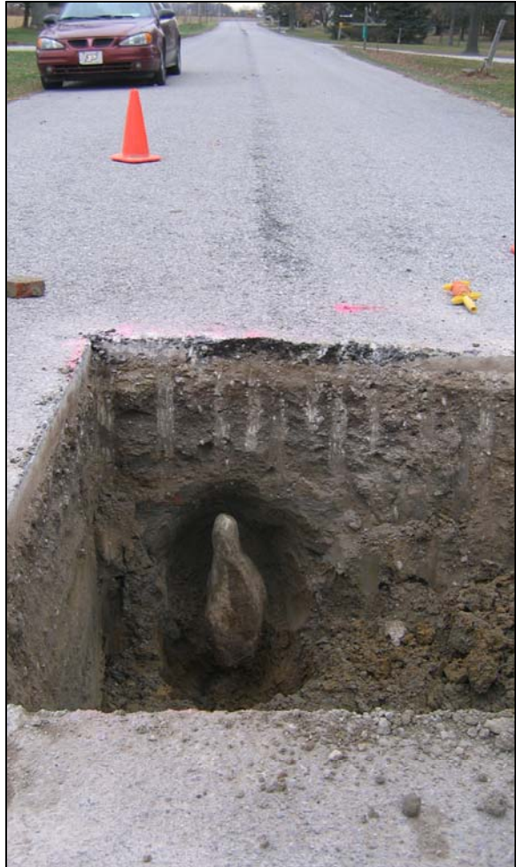
Corner stone. View from east of fully exposed stone and County Road 700 South to the west.
