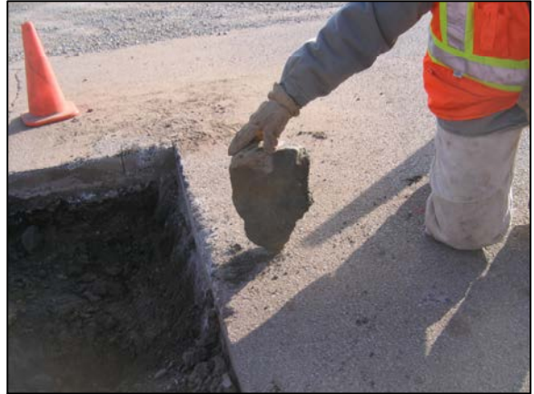
The stone temporarily removed from the road bed, showing its shape with a pointed bottom.
