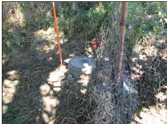
The harrison monument set in place of the top stone and over the bottom stone.
