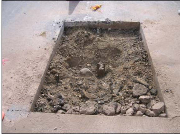
View of the stone as first exposed, along with the railroad rail.
