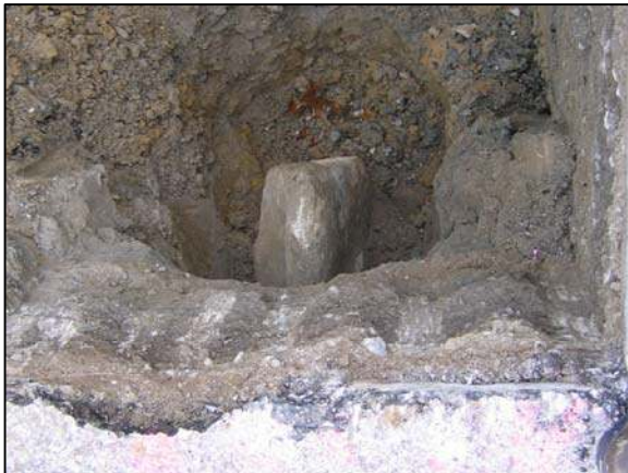
Corner stone. View from above.
