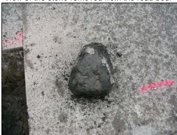
View of the stone removed from the road bed.
