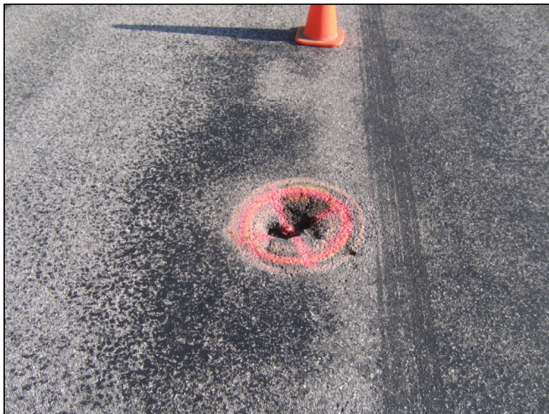
View of the bolt spike found prior to excavation.
