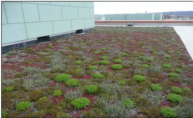
Figure 1 Vegetated Roof, Washington, DC (USEPA, picasaweb)
