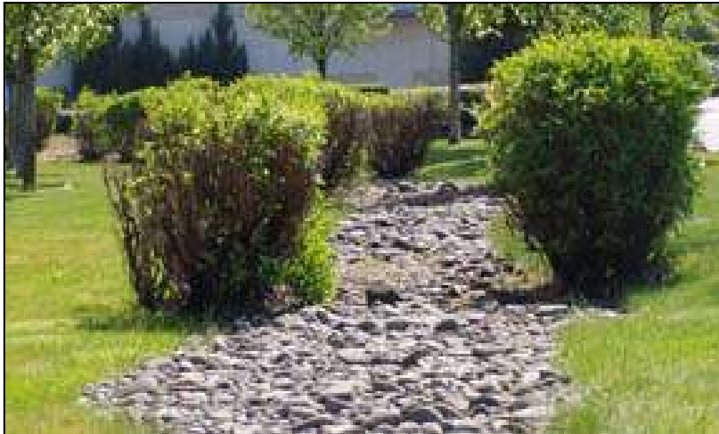
Figure 1 Gravel trench directing water from the parking lot to a vegetated filter strip in Springfield, OR (Springfield Environmental Services Division)
