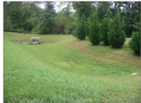
Figure 2 Dry Pond: Photo courtesy of Fairfax County VA Department of Public Works and Environmental Services.
