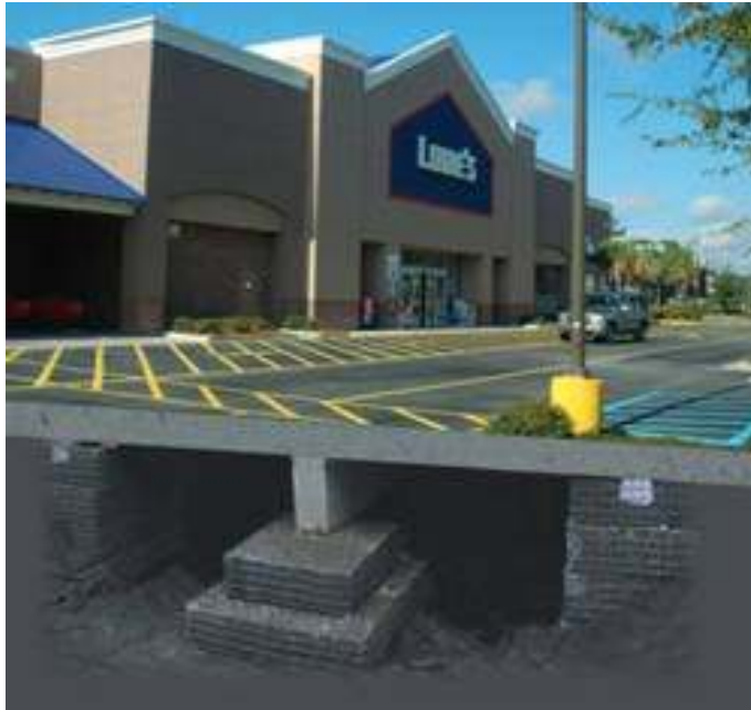
Figure 1 Photograph courtesy of Vertex Design Group
