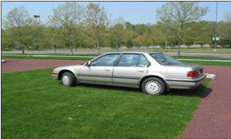
Figure 1 Grassed overflow parking areas (NEMO, University of Connecticut)
