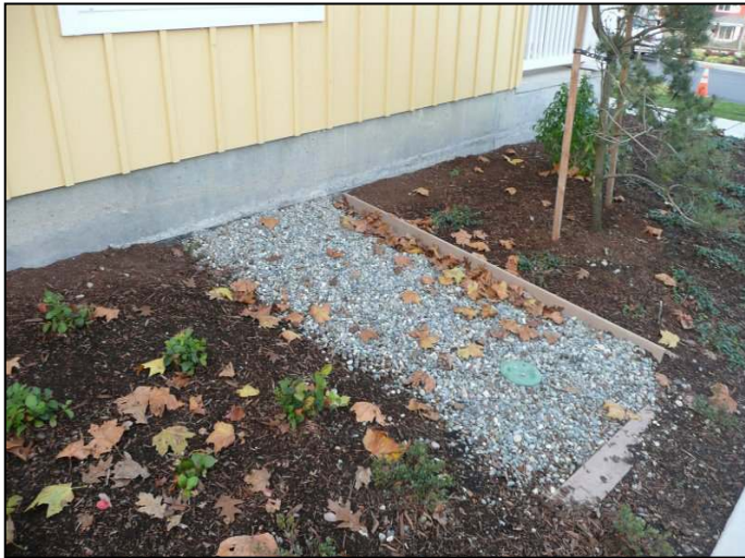
Figure 1 Infiltration Bed, Seattle, WA (USEPA, picasaweb)
