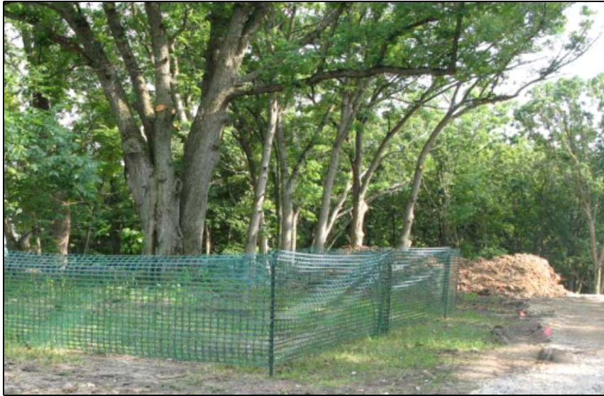
Figure 1 Areas where heavy equipment is not allowed are fenced off to avoid compaction of soils and damages to vegetation (MD Custom Homes, WI)
