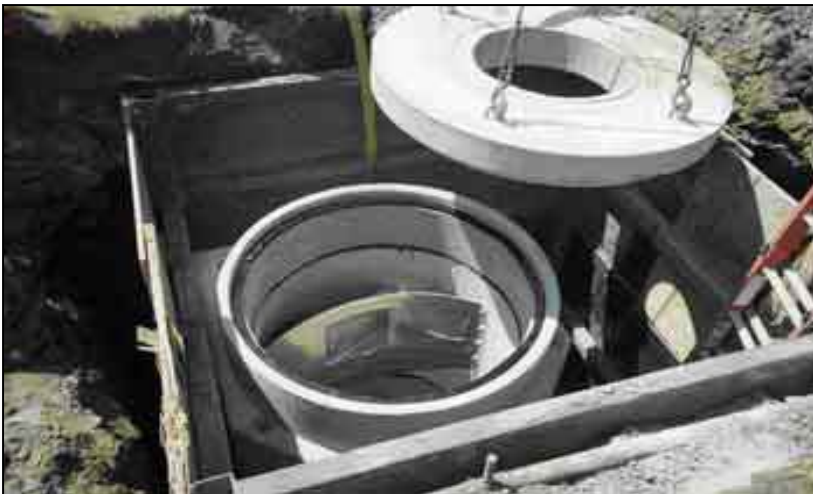
Figure 1 Installation of hydrodynamic separator (Johnson County, Kansas Stormwater Management Program)
