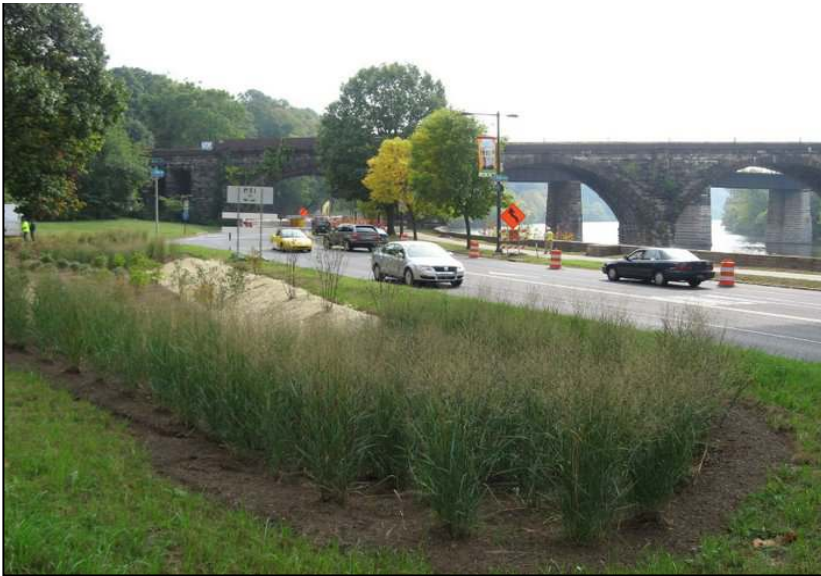
Figure 1 Vegetated Swale, Philadelphia, PA (USEPA, picasaweb)
