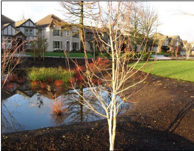
Figure 1 Pond collecting runoff from rooftops, sidewalks, and yards, Wilsonville, Oregon (USEPA, picasaweb)
